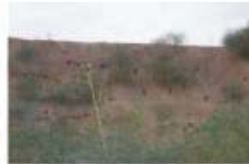
9. These are exposed soil surfaces due to soil erosion. The black holes are nests of birds like Parrots ( Psittacines ).
